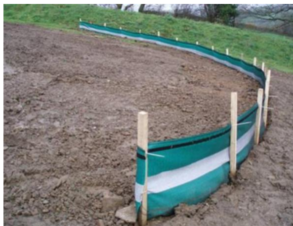
Figure 6-1: Examples of suitable silt fence mitigation ensuring maximum safeguarding efficiency
